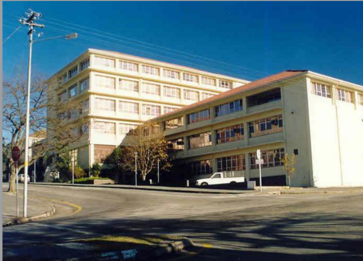
The old Biological sciences building cannot accommodate the rapid increase in research priorities of the University
